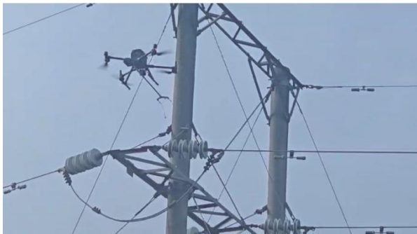
Inspecting tension insulator strings
