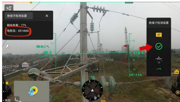
Drone captured footage (tension string)
