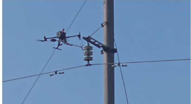
Inspecting suspension insulator strings
