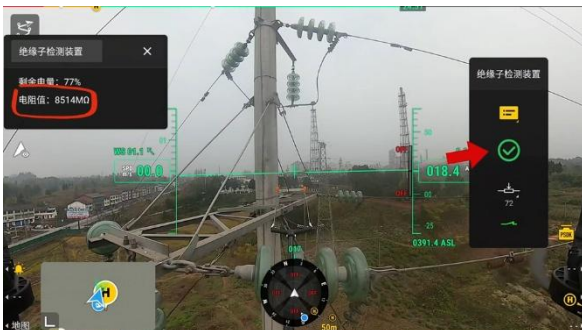
Drone captured footage (tension string)
