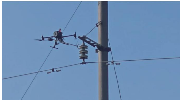
Inspecting suspension insulator strings
