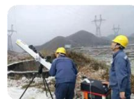
Laser Cannon De-Icing : High power consumption, small range
