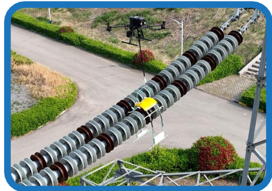
Mounting the robot
