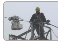
Robotic Mechanical De-Icing: It is difficult and highly dangerous to install robots on iron towers after they have iced up.
