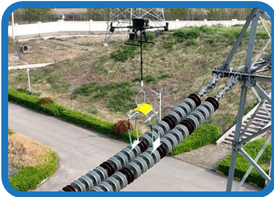
Mounting the robot
