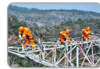
Direct Current De-Icing: Operation is complex and energy consumption is high.
